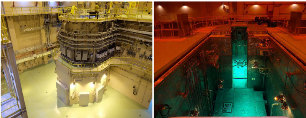
The JRTR facility has advanced design and capabilities in the region.
